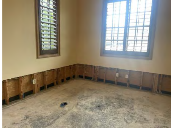
Typical interior (Photo Taken on July 21, 2022)
