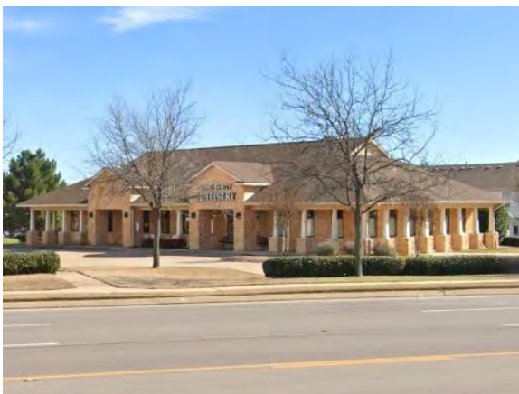
Lease Comp #5 6248 Davis Office
