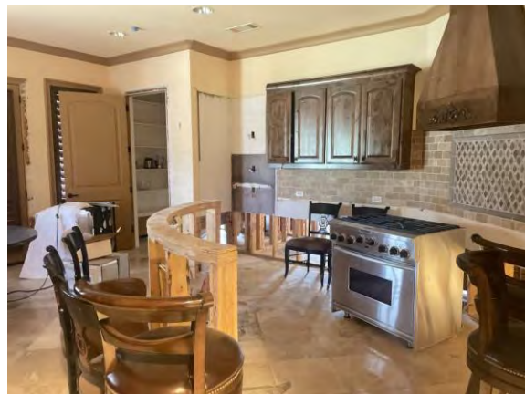
Typical interior (Photo Taken on July 21, 2022)
