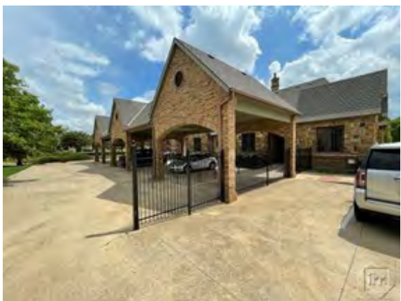
Rear gated entrance and covered parking for tenants
