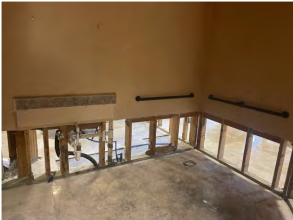
Typical interior (Photo Taken on July 21, 2022)
