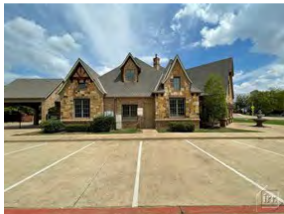
Side View - Exterior
